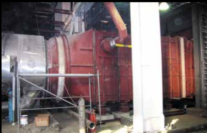
Round and Rectangular fabric expansion joints for a GT application in Moscow
